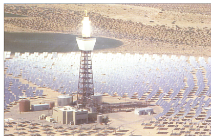
Fig. 3.2 Solar Two in operation at Barstow
